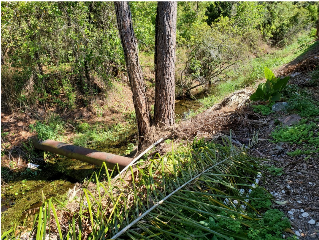
This picture depicts the City water main crossing of the ditch.
