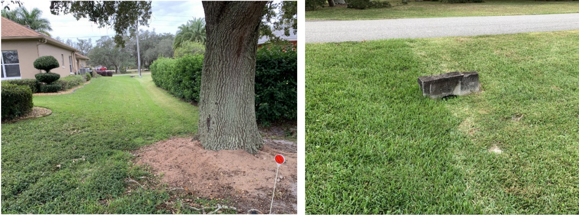
Pictures of Culvert Crossing and Side Ditch from Previous Report
