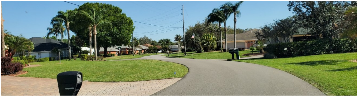
This is the view south along Lost Ball Drive. Main area of concern is on the right of the road. The ditches appear to be fairly shallow and may have some undulations.
